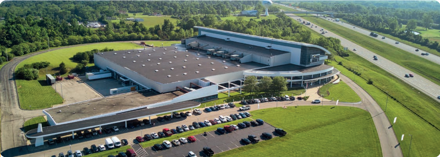
Modula Plant – Franklin, Ohio
