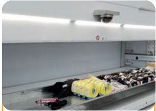
External Bay Lighting
